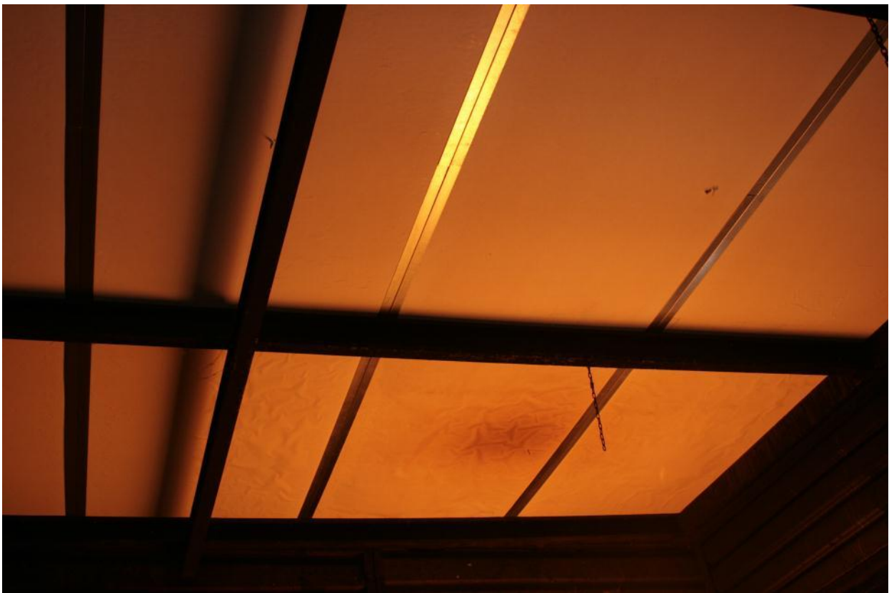
Figure 4.1.6: Note discoloration starting above fire source area
