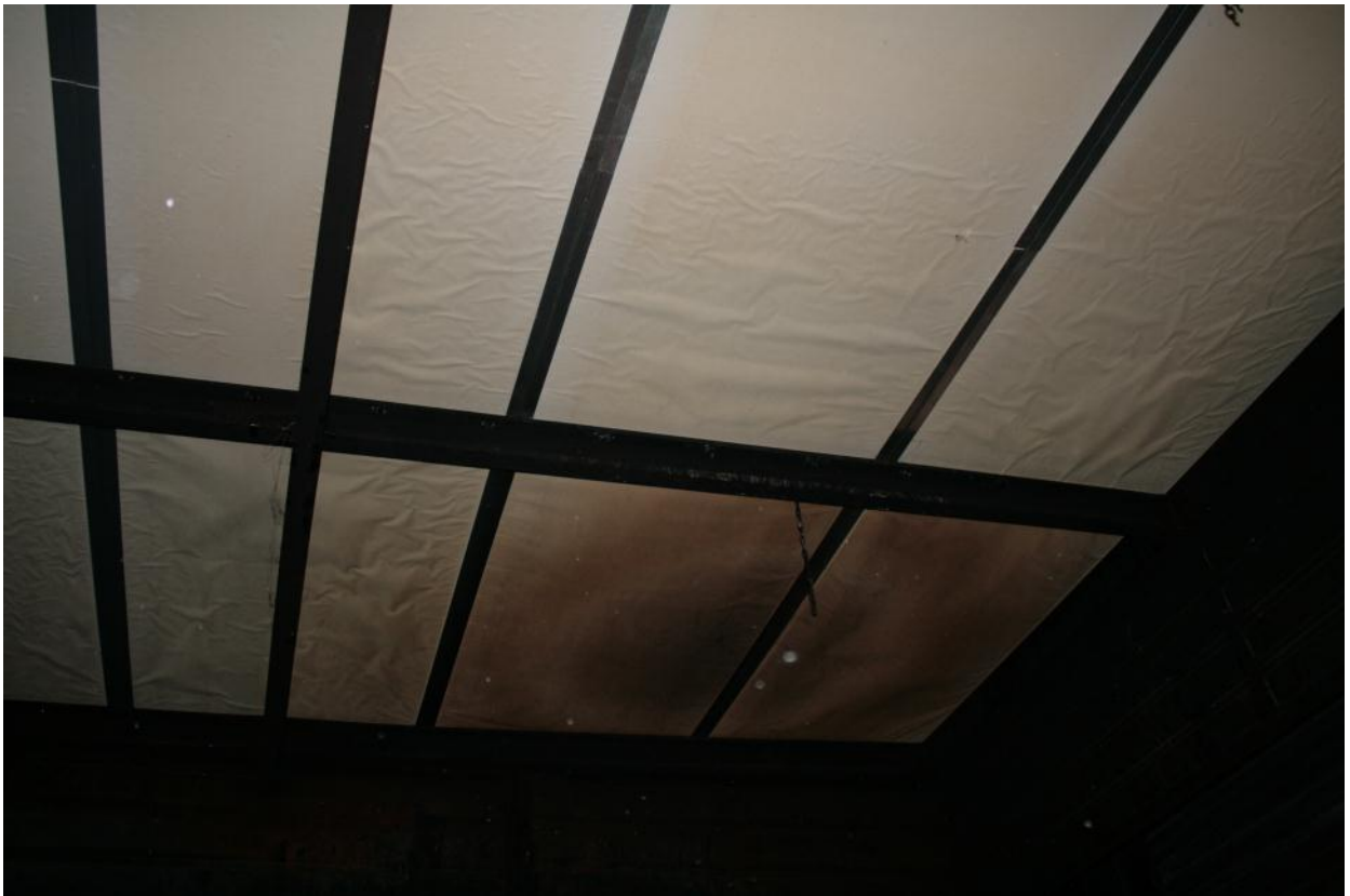
Figure 4.1.10: Test installation subsequent to completion of the test
